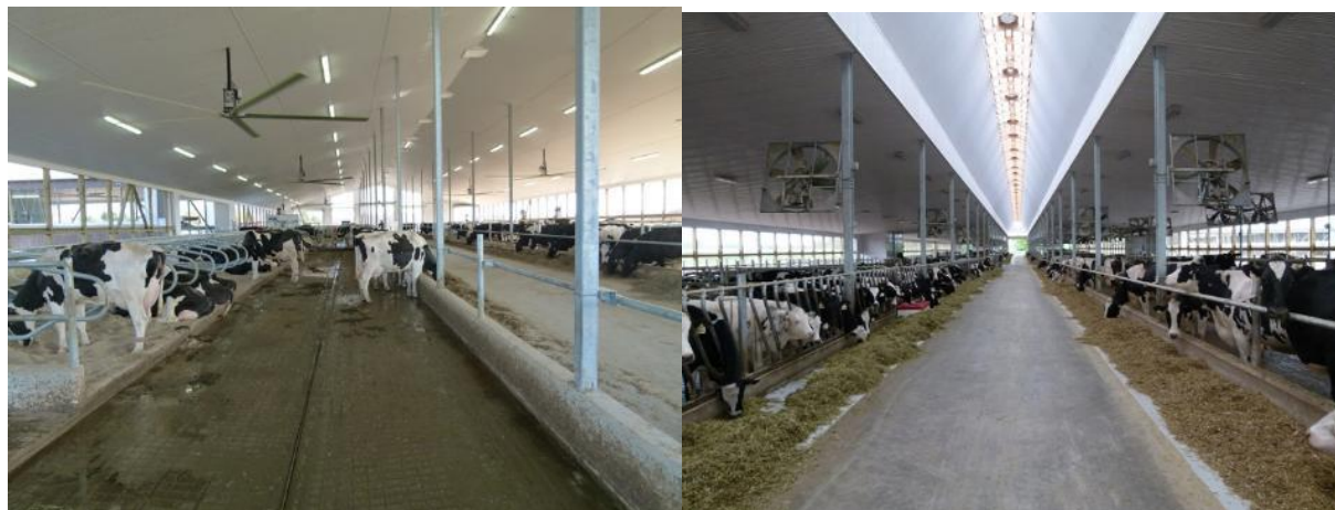
FIGURE 13. HIGH VOLUME LOW SPEED FANS (LEFT) AND HORIZONTAL FANS (RIGHT).
