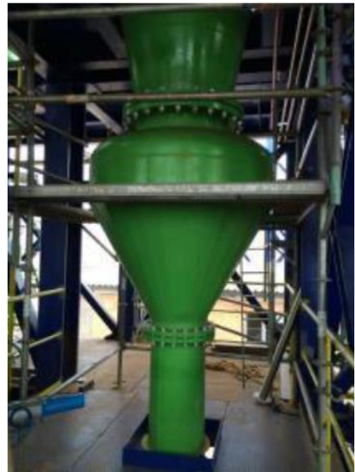
Figure 13: Cyclone precipitator.
